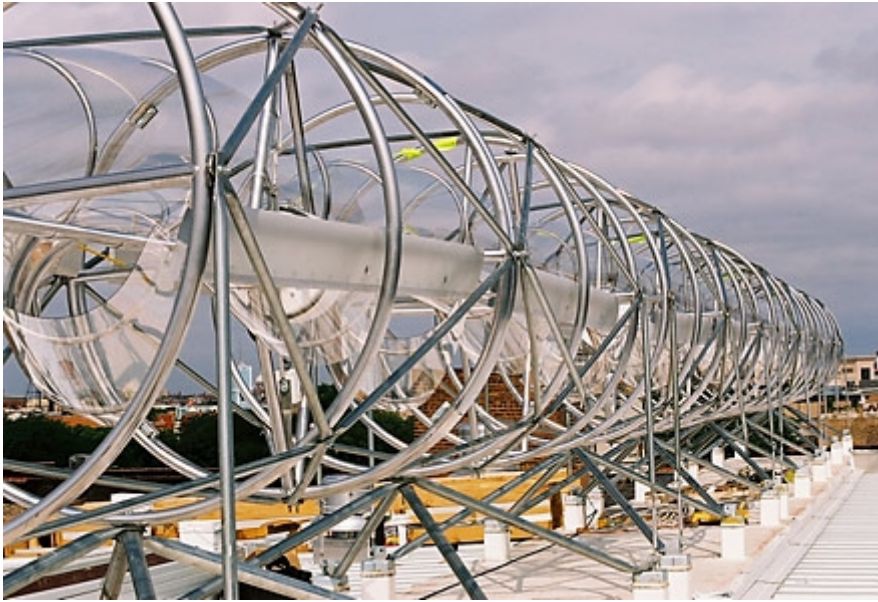
The wind turbine on top of the Near North SRO. Photo by Kurt Holtz.
